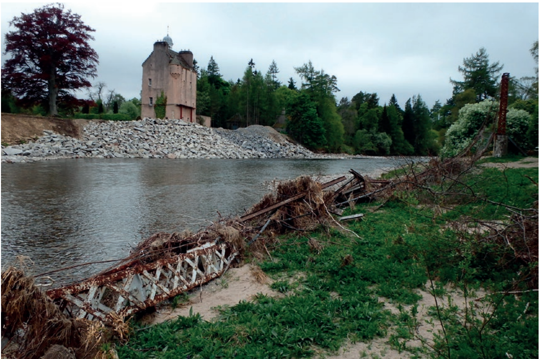
Figure 3. Collapsed Abergeldie Castle Suspension Bridge from the River Dee winter spate of 2015-16
